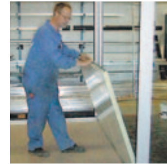
Simple assembly of wall panels
